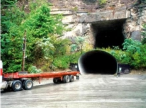
Front Chamber Entrance
